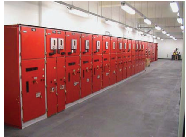
Fig. 8 Air-insulated switchgear 8BK, 6.6 kV, with 7SJ63-protected and controlled circuit-breakers
