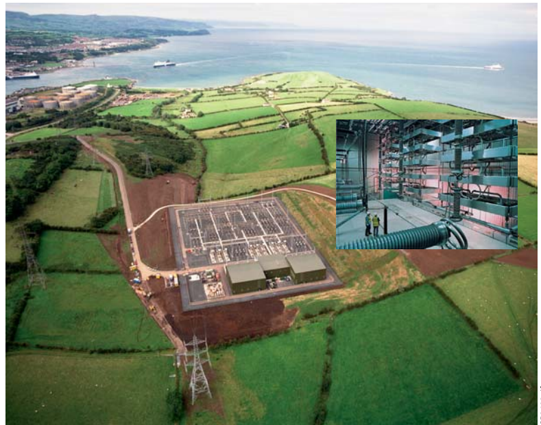
Fig. 1 HVDC power station in Ireland
