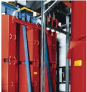
4.9-MVA GEAFOL static converter transformers for a gold mine in South Africa 1700 m below ground at an air humidity of 90%.
