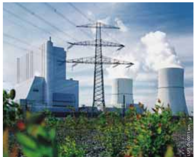
Fig. 1/13 SIPROTEC 4 application in power stations
